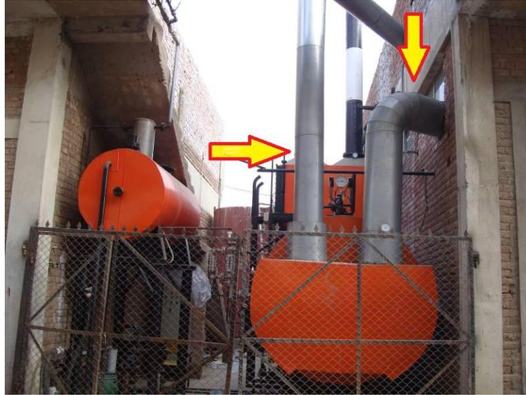
Figure 3: Waste Heat Channels from Generators to WHRB
