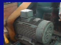
Variable speed Drive
